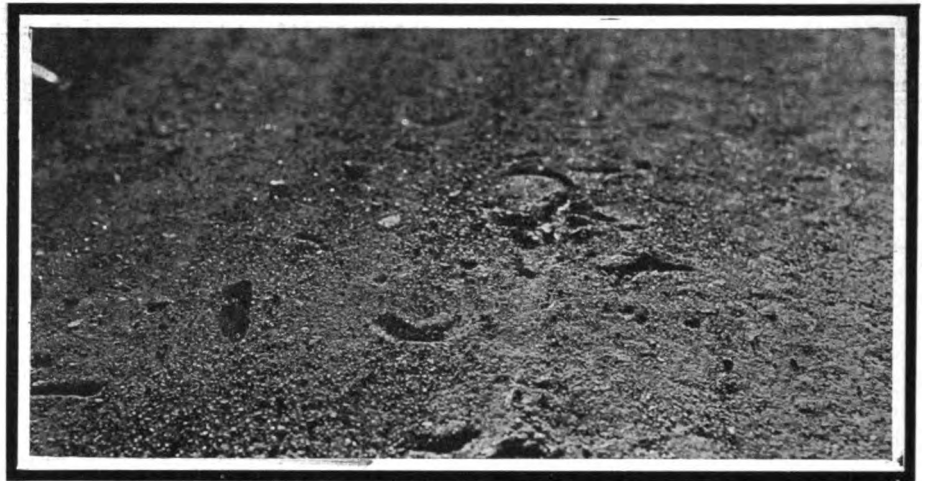
When the horseshoe calks penetrate the macadam, the end of the road is in sight:
